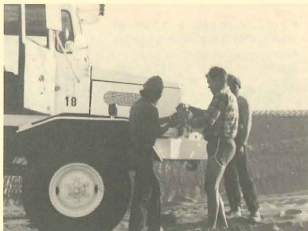
Vibrator mechanic, Scott Netzer, and labourers repair vibrators.
