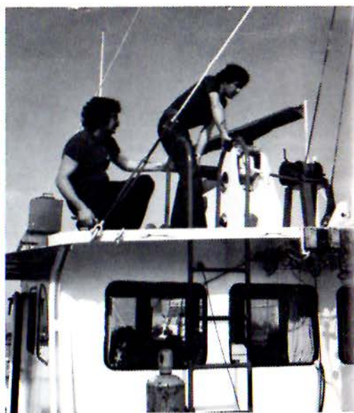
Two of the ship's crew preparing to install some communication equipment.
