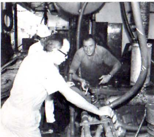
Bill Blakeley (L) and Pete Reichle inspecting compressor engines (shipyard foreman in background).
