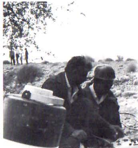
Shooters setting off dynamite charge.
