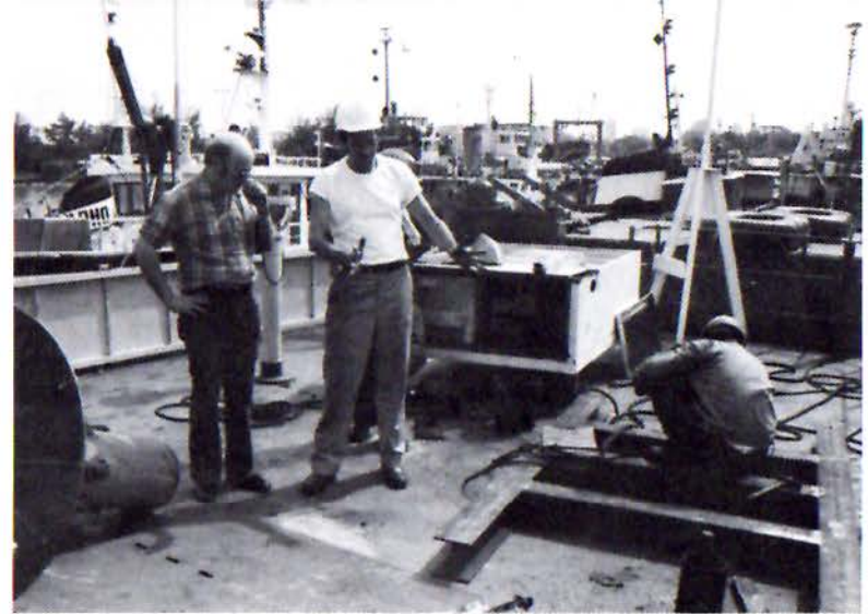
Eric Jones (L) and Lorton Trent discussing installation of MARISAT.
